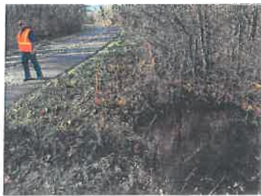
Collapsed 60” CMP on Wolfrum – Spring 2022
