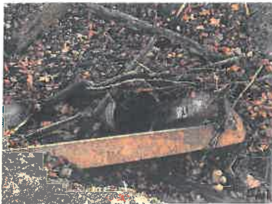
Collapsed 60” CMP on Wolfrum – Spring 2022
